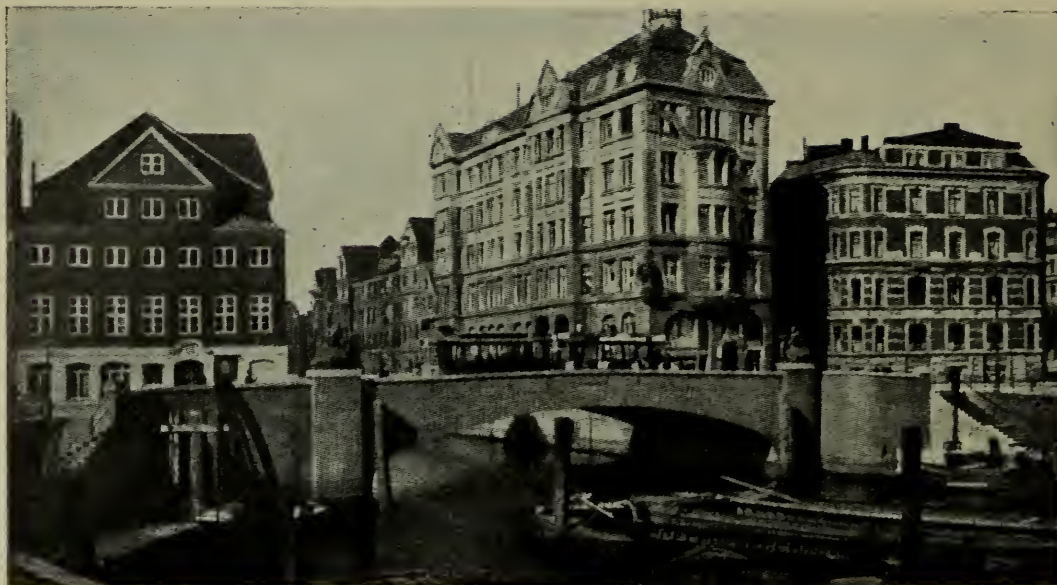
FIG. 5.—SCHAARTOR BRIDGE AS COMPLETED.
